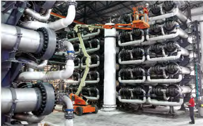
High flow. This reverse-osmosis plant in Ashkelon, Israel, will eventually turn out 100 million cubic meters of fresh water a year.
